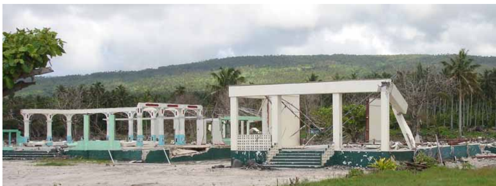
Tsunami damage in Samoa
